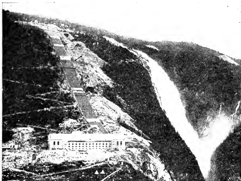
FIG. 65.—Large Hydro-Electric Power Station at Rjukan, Norway, Showing Ten Five-foot Penstocks and Method of Anchoring Same.
